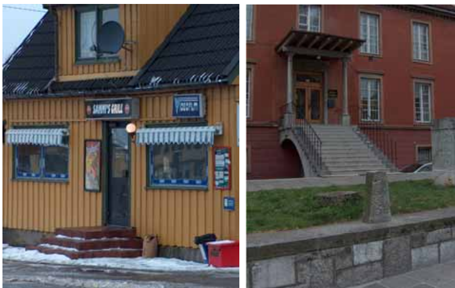
Figure 1. Achieving level access to premises in existing and sometimes narrow city streets is no easy task. (Left, Råde, Norway; right, Ljubljana, Slovenia)
