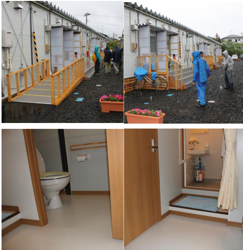
Figure 3. Ramp and flat deck type entrance and gentle stairs type entrance (Upper two). Flat access toilet and step to bathroom (below two)
