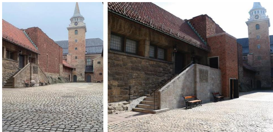
Figure 5. L.h.s.: The courtyard before intervention. R.h.s.: An elevator tower has been established in connection with the new stair. (Photo 1: Arkitektskap AS; 2: M. Brenna)
