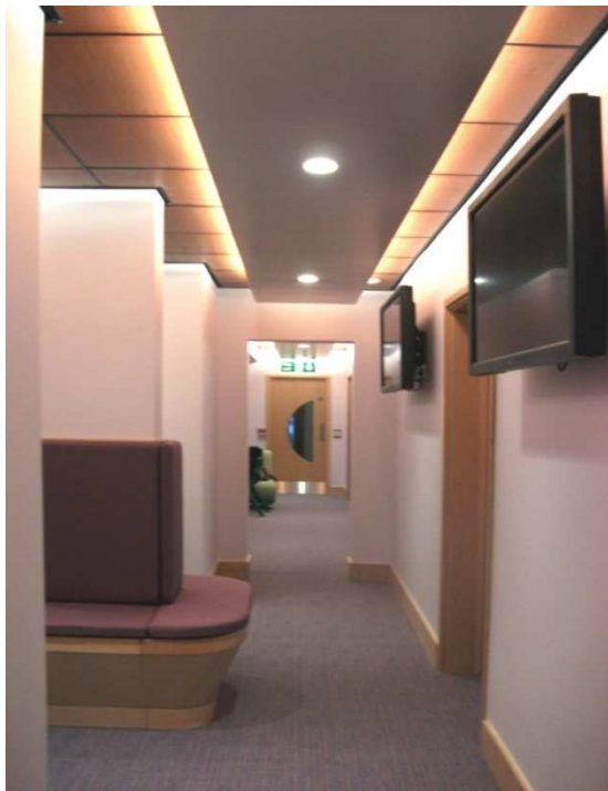
INDIRECT PERIMETER LIGHTING
