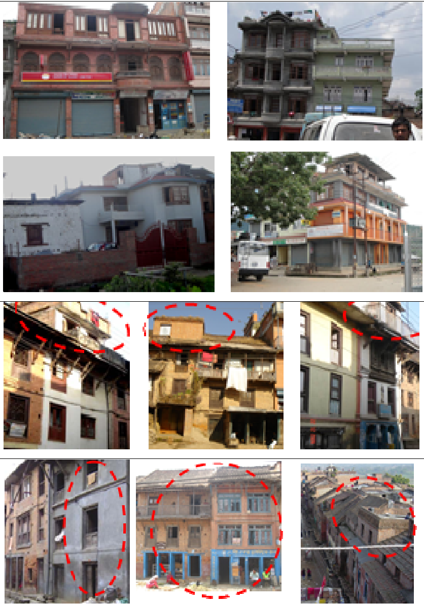
Fig. 4.3. Transforming traditional newari houses – uses and density
