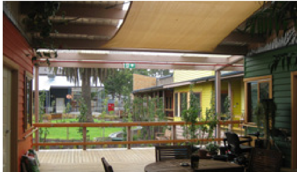
Fig.7 Potter Street Redevelopment, Dandenong, Australia. Sheltered outdoor area outside bedrooms, view to garden. Allen Kong Architect, Honourable Mention. Picture: Allen Kong
