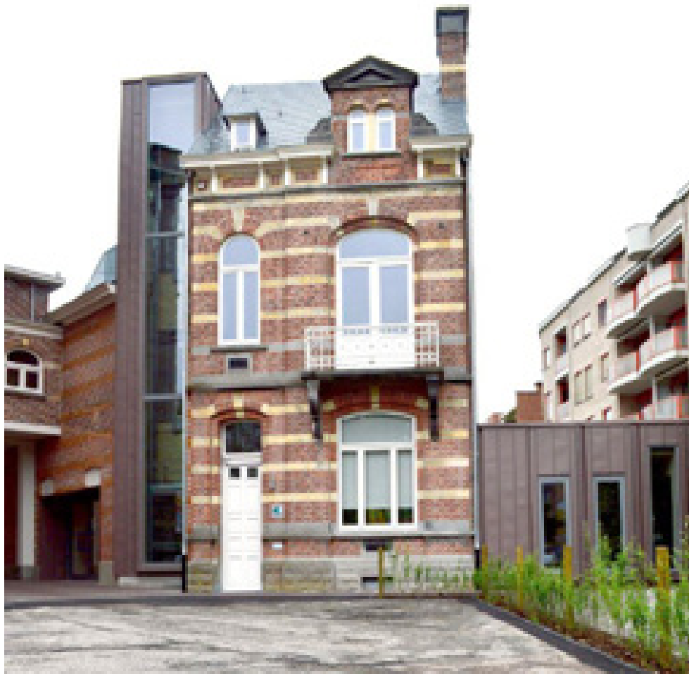
Fig. 1: Façade renovated porter's lodge
