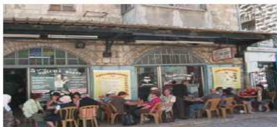
Existing awning - support location according to the opening, arch and upper balconies structures. Bogod-Krendal -Niv Design
