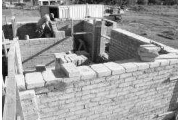
***LMI-1 Prototype, Series 012 Universal Home™ design- Abilene, Texas. First HUD funded Lime stabilized Compressed Earth Block Home in US History. Constructed in 2010. COURTESY PHOTO***
