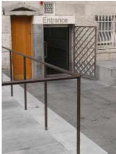
New entrance - http://www.hkengineering .ie/?page_id=30
