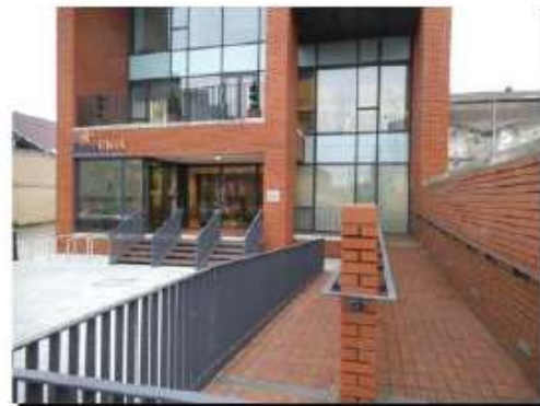
Access ramp to main entrance
