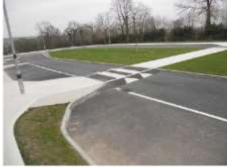
Set Down Area at side of Building
