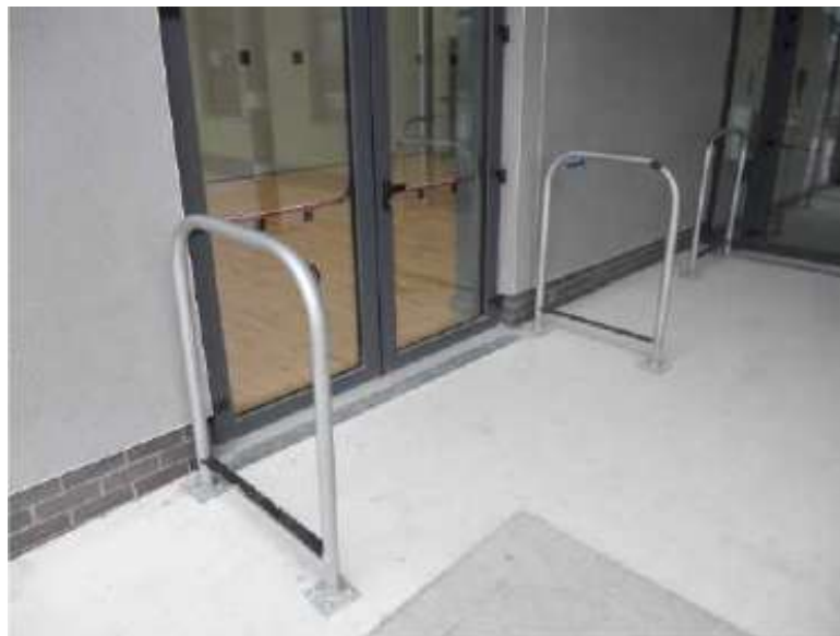
Railings outside of doors. Note to the bar at bottom for cane users
