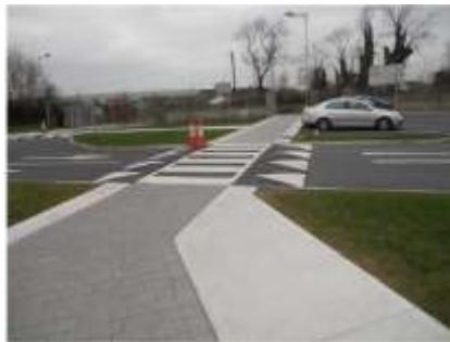
Level Crossing near entrance
