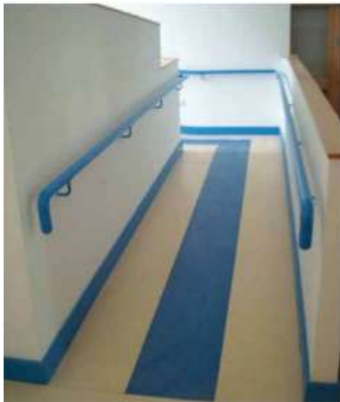
Colour used on floor, to aid circulation of building
