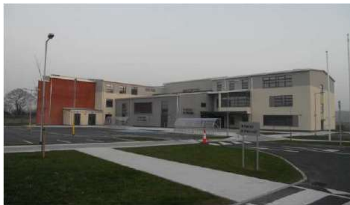
Front of Building and Car park
