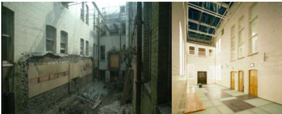
Cork Courthouse Progress Photography 30 May 2003 Ref: 10
