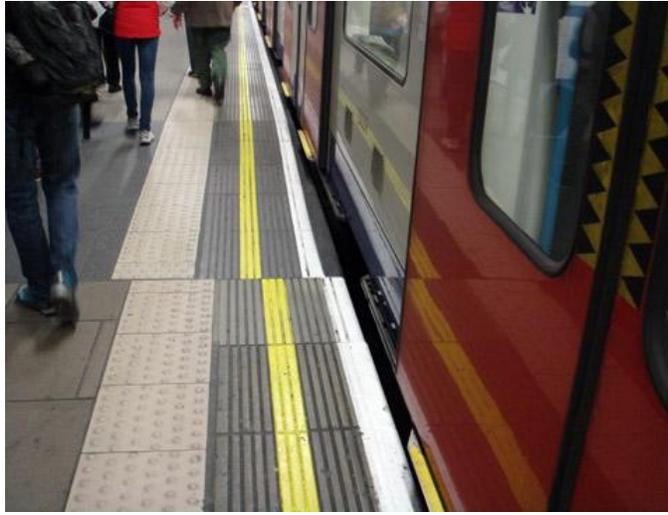
***Figure 3 : Raised platform (hump) in the London tube (Metadyne).***
