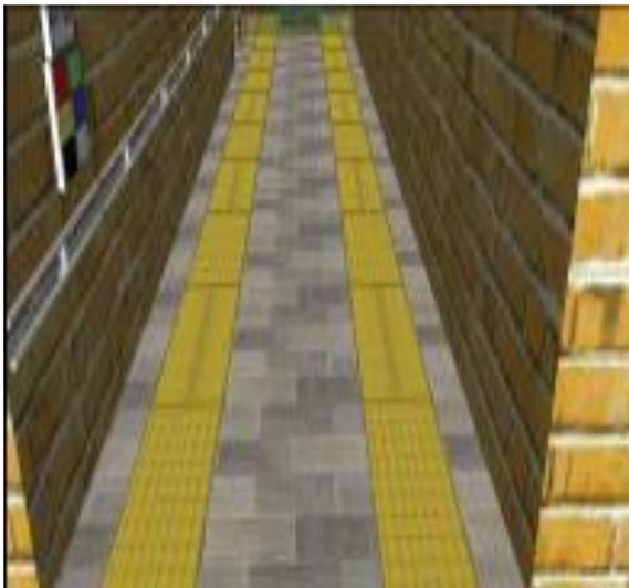
*Fig 6.2: tactile tiles as the flooring material*
