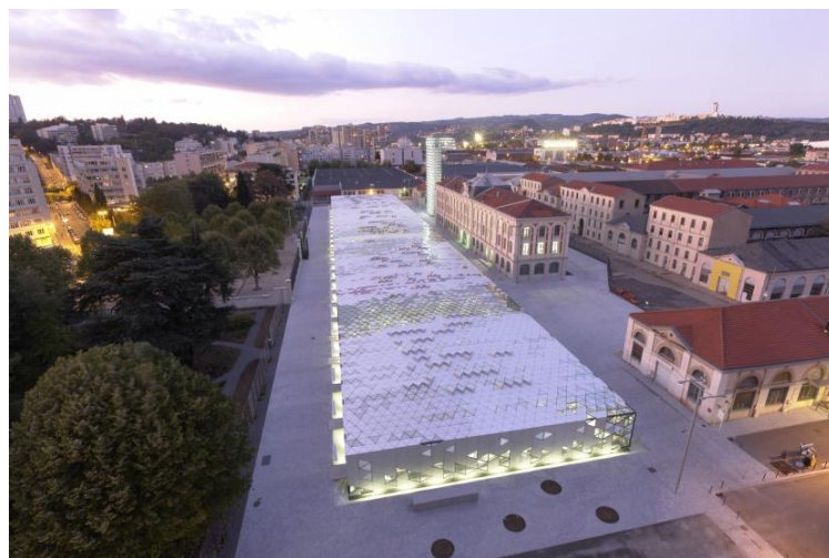
Saint-Etienne Cité du design buildings - ©LIN agency
