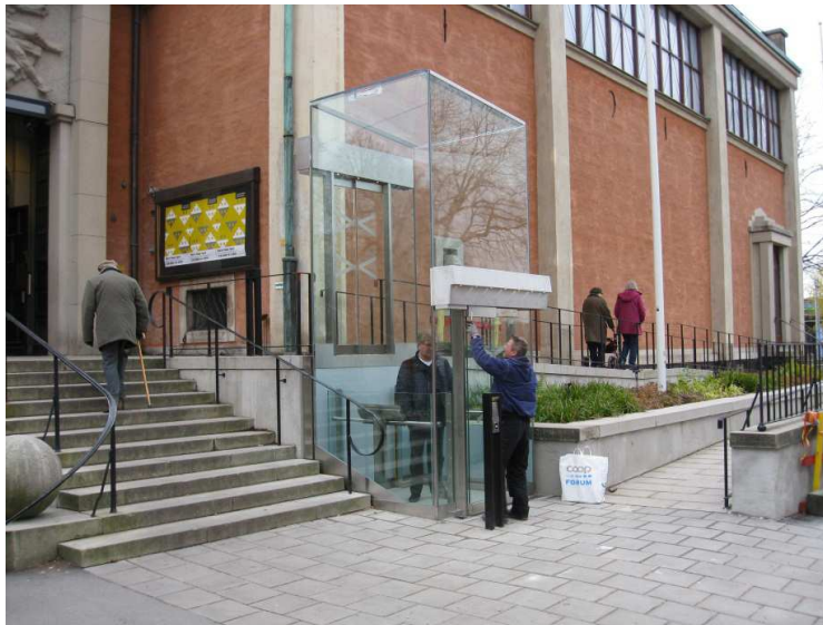
The Liljevalchs Art Hall after completion of the work, with a new ramp and a new lift solution
