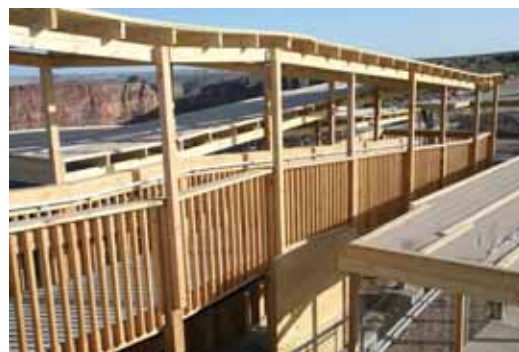
The temporary ramp when it was first inaugurated
