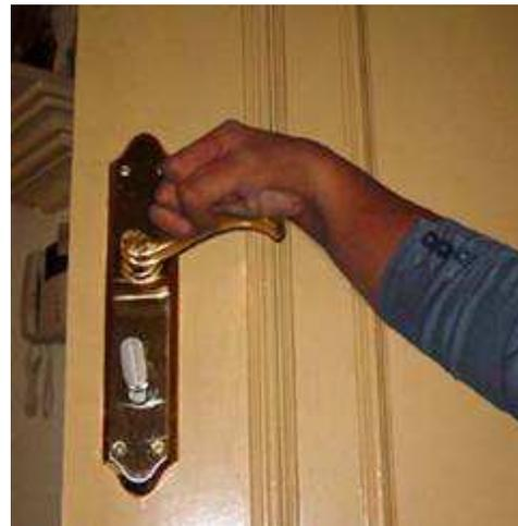
*A lever handle can be used with limited dexterity*
