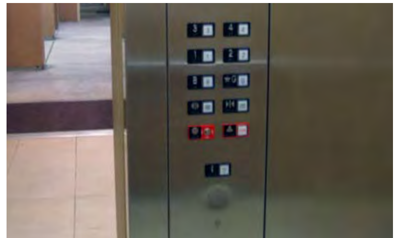
The elevator buttons have both braille and raised letters for people with visual impairment.
