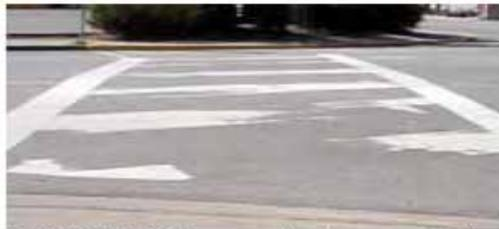
(IMAGE 3) Crosswalk does not line up with the curb cut
