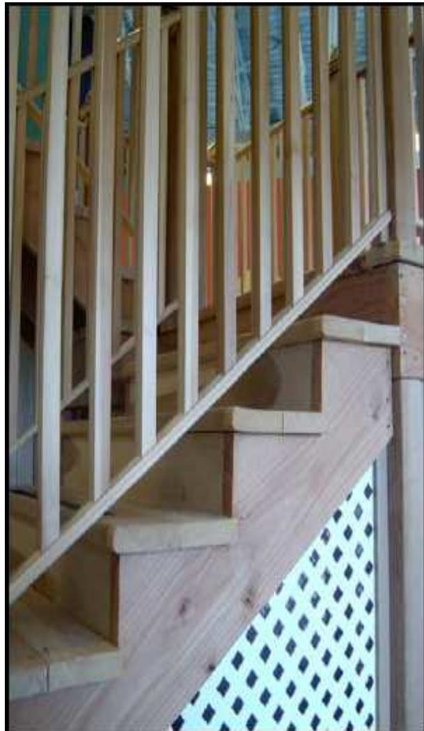
tread creates a larger target to increase foot accuracy. A child height railing (at a maximum of 28
