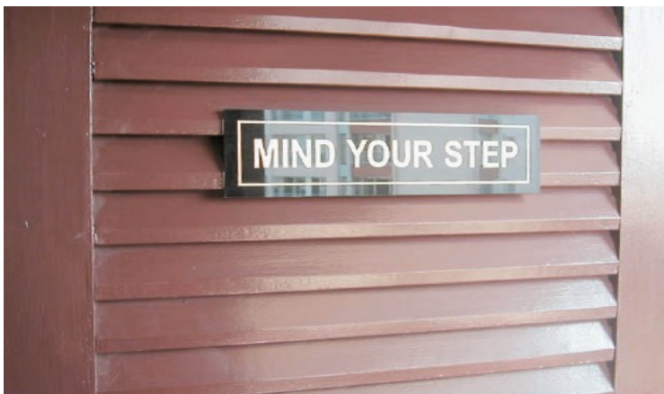
Fig 3. Although the sign provides a warning, it also demonstrates a weakness in the design.
