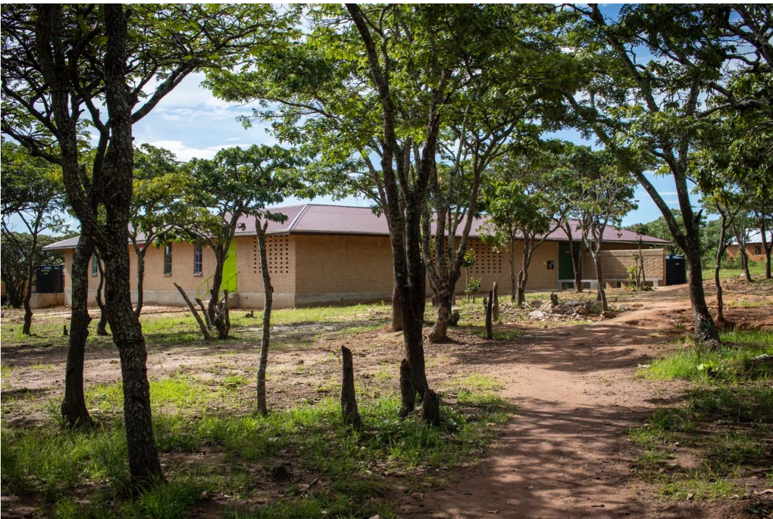
The buildings are built in Interlocking Stabilized Soil Blocks that are easily produced by the village using local clay. Photo: James Kasela
