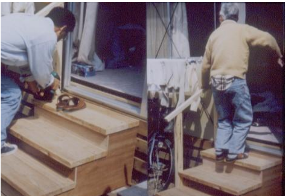
Figure 2. Inverted U- shaped gutter placed at the entrance of emergency temporarily house (upper photo from Kobe city website of archives). Easy steps made by volunteers, and resident tried up and down frequently (below)
