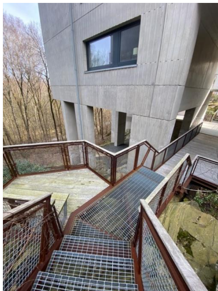
Figure8. Staircases composed of steel grids. Figure 9. The natural ground is sometimes integrated in the system of stairs. (Photos: Ida Sandström)
