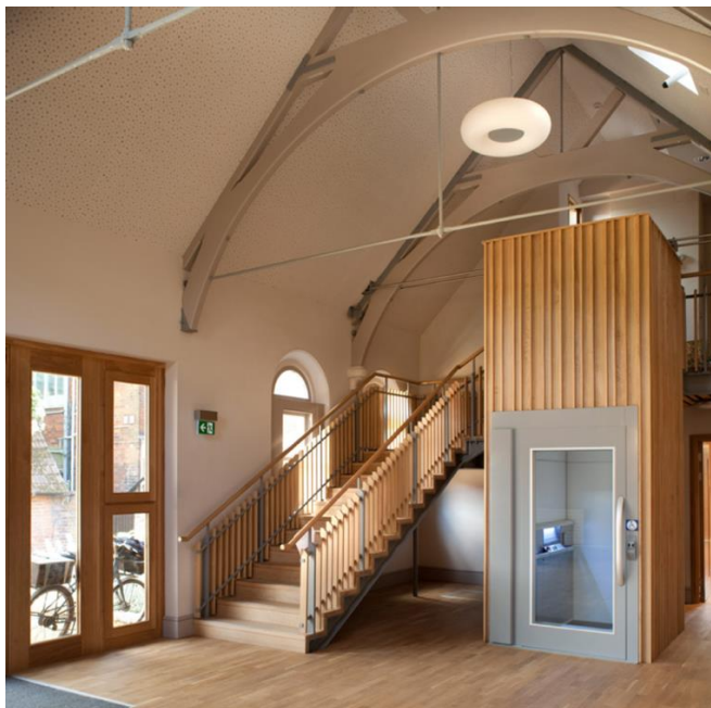
Elevator and stairs added later
