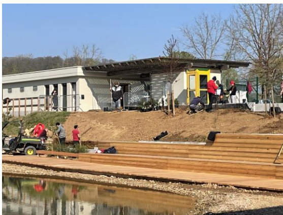
Image 4.-Construction of smooth ramp
