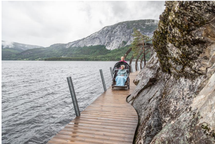
Image 2.- A suspended path over the lake. "We want as many people as possible to be able to get out into nature, not just the most active people", Aslak Momrak-Haugan, Project Manager.
