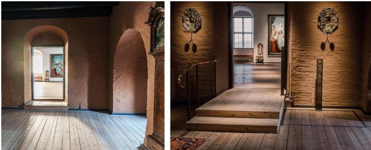
Figure 3. L.h.s.: One of the halls before intervention. R.h.s.: A lifting platform is integrated in the floor. (Photo 1: Oslo Byggentreprenør AS; 2: A.M. Malkenes Mathiesen/The Norwegian Defense Estates Agency)
