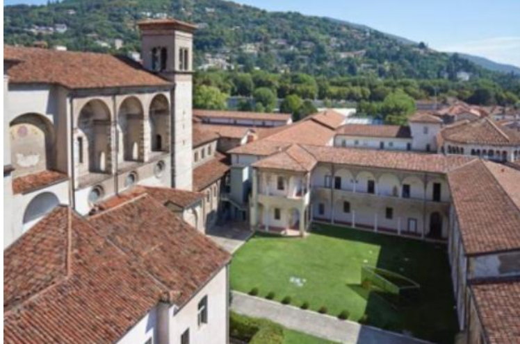
Figure 2. Santa Giulia Monastery, aerial view
