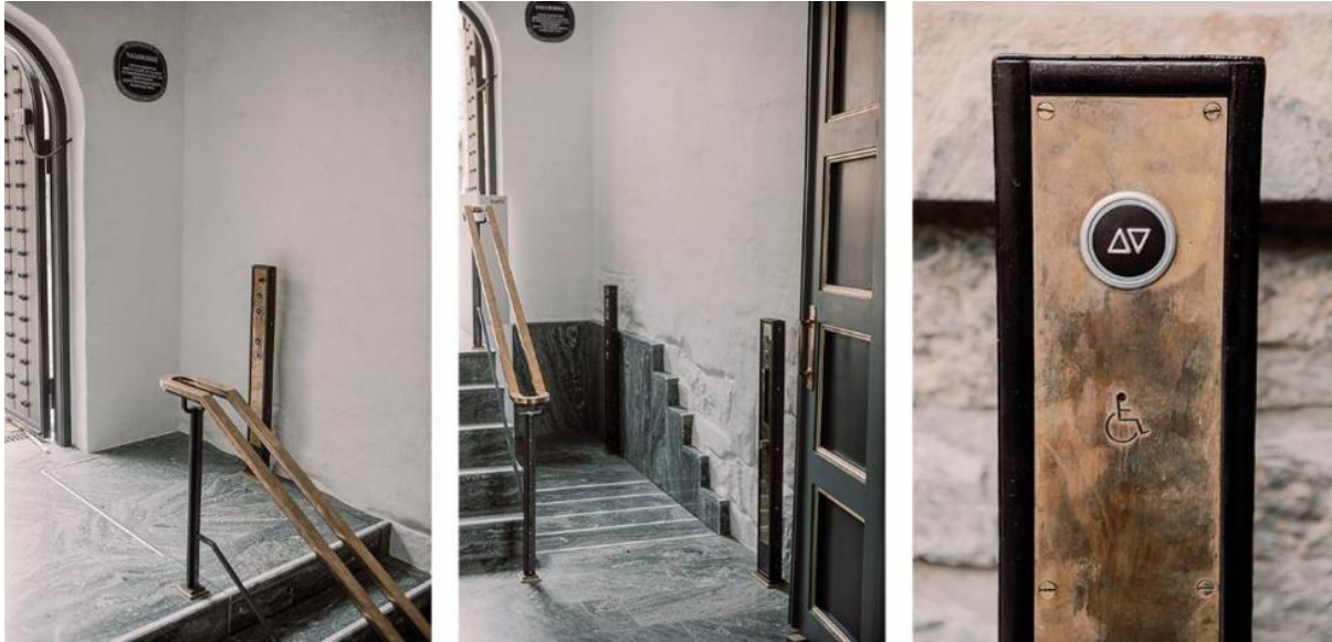
Figure 7. A lifting platform is integrated in the stair in the church's entrance hall. (Photo: Anne-Margrethe Malkenes Mathiesen/The Norwegian Defense Estates Agency)
