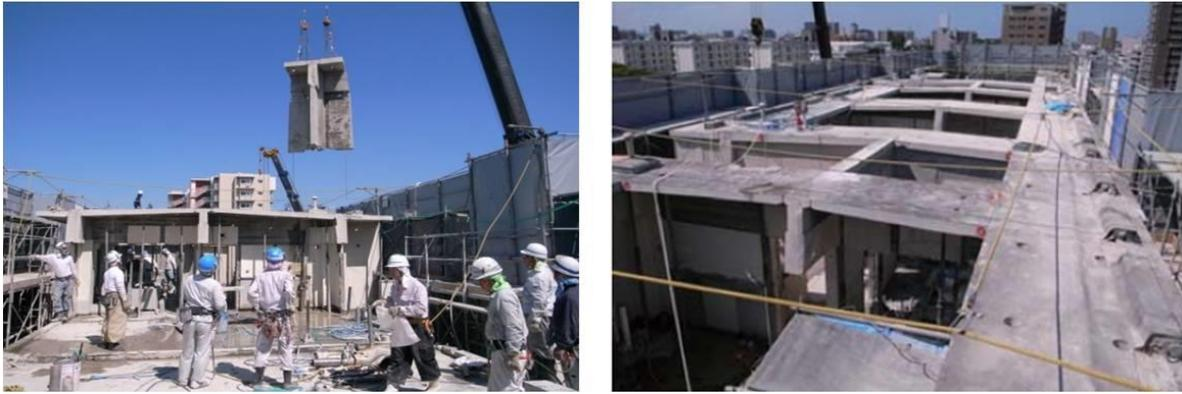
**Figure 8: Cutting process to remove upper levels**
