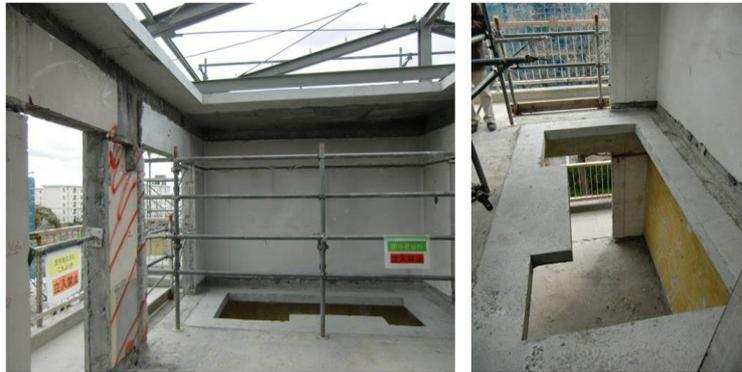
Figure 6: Slab cuts to join apartments and install inclined roofs
