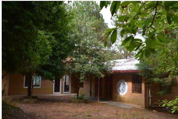
Image 1: Front view of Building 1 and 3
