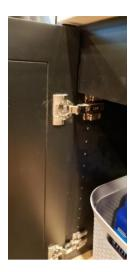
View of easy release base cabinet hardware that allows for quick removal of base cabinet doors underneath both sinks and induction cooktop.
