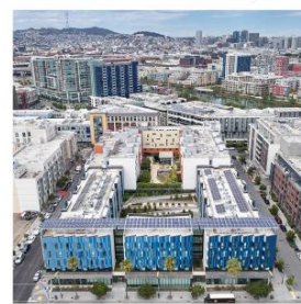
The Edwin M. Lee Apartments is San Francisco's first integrated veteran and low-income family housing development.
