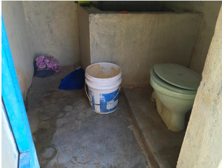
Picture 9 Some persons with disabilities have retrofitted western water closets. A water storage tank is constructed behind the water closet.
