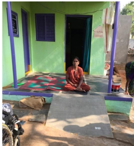
Picture1 All houses are built on a plinth a foot or two high.
