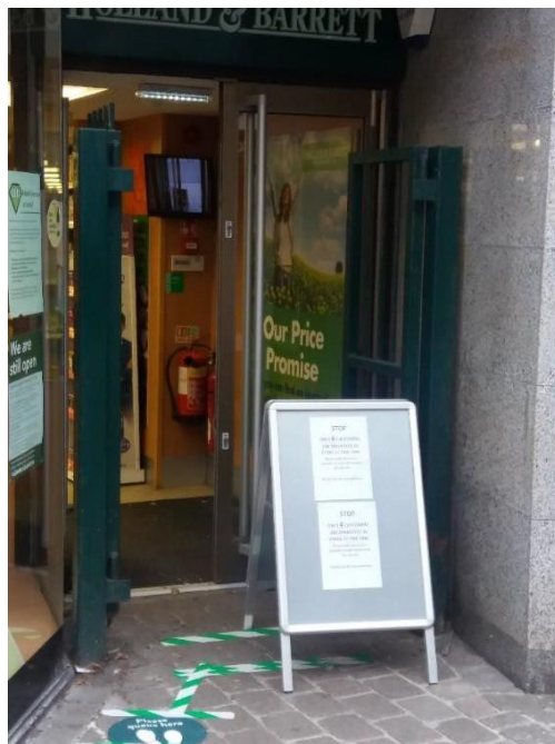
Figure 2 –Difficult entry hazardous for disabled people
