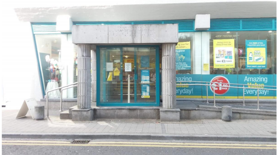
Figure 4 – Ramp in, stairs out is common place, with no allowance for wheelchairs
