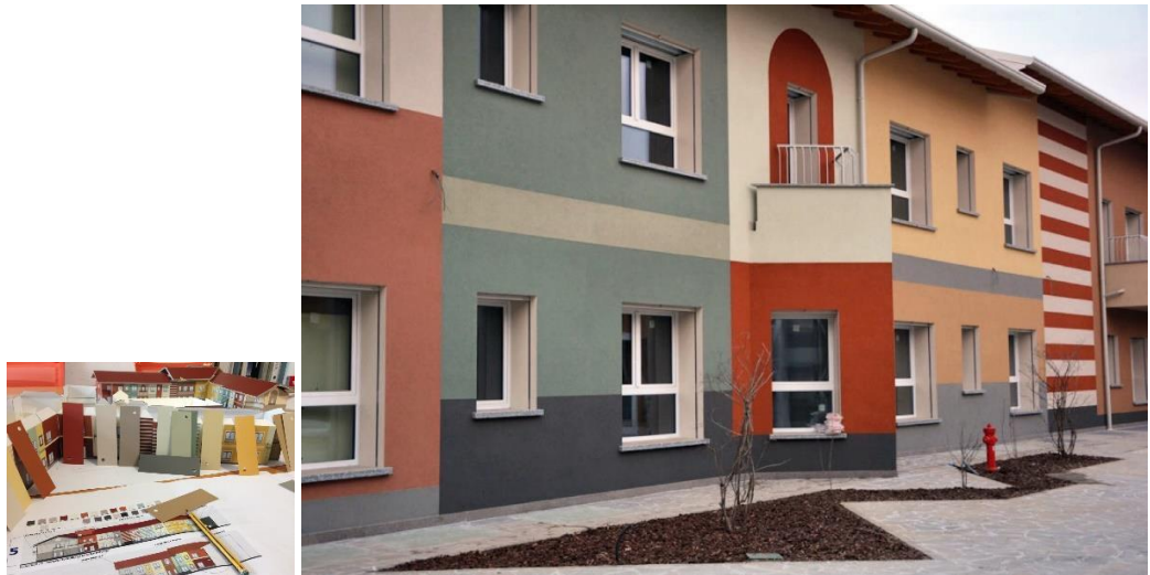
Figure 9-10 – Alzheimer's village "The Rediscovered Country" of Monza (Province of Monza Brianza): the different colours used for the facades of the buildings
