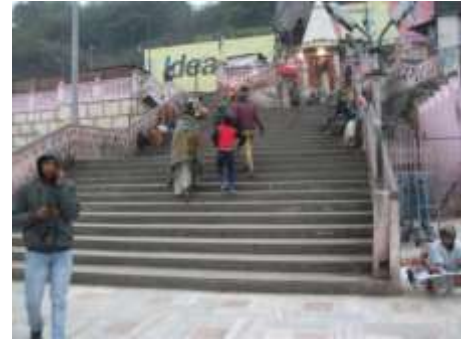
Figure 8 Staircase joining Ghat and Major Street. Riser is 17cm, run is 38 cm, height of side rail is 1 m. (Source: author)
