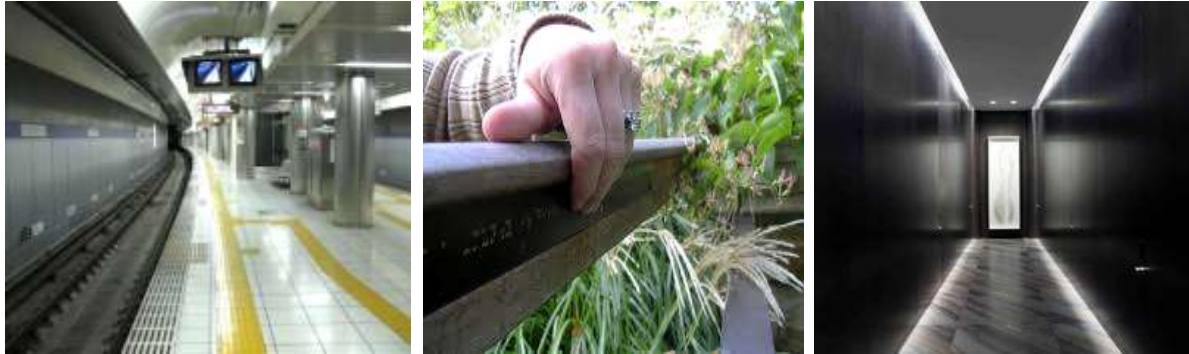
Figure 5 Guide paths: (a) Tactile tiles (b) Handrails with Braille (c) Guiding light strips (Source: http://en.wikipedia.org/wiki/Tactile_paving , http://www.dev.ihcdstore.org/?q=node/130 , https://www.pinterest.com/geochevez/hallway/ )
