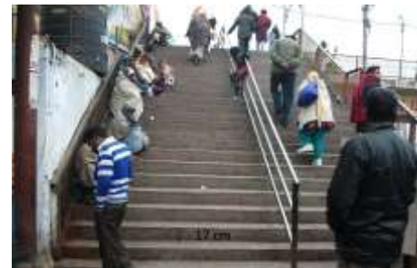
Figure 9 Representing one of the staircases of an important bridge. Riser is 17cm and runner is 27 cm. (Source: author)
