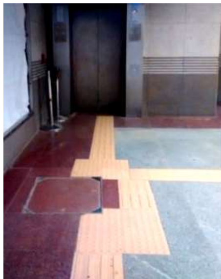
Figure 7 Adjustment with tactile tiles junction design
