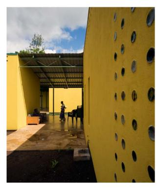
Large covered open air areas allow natural ventilation and free air movement within the building, providing shade and protection from rain. Covered outdoor spaces are used for meetings and seminars. photo: Juha Ilonen
