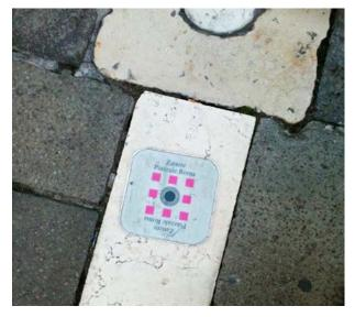
Audio signage in Venice for tourists works greatly for visually-impaired and with the devices of the hard of hearing. The technology integrated in the paving is not disturbing the historical environment. In Venice, there is an ancient way-finding system for pedestrians hidden in the paving: tiles in one direction are meaning direction San Marco (S. Marc Square) and in the other way the perpendicular "calles".
