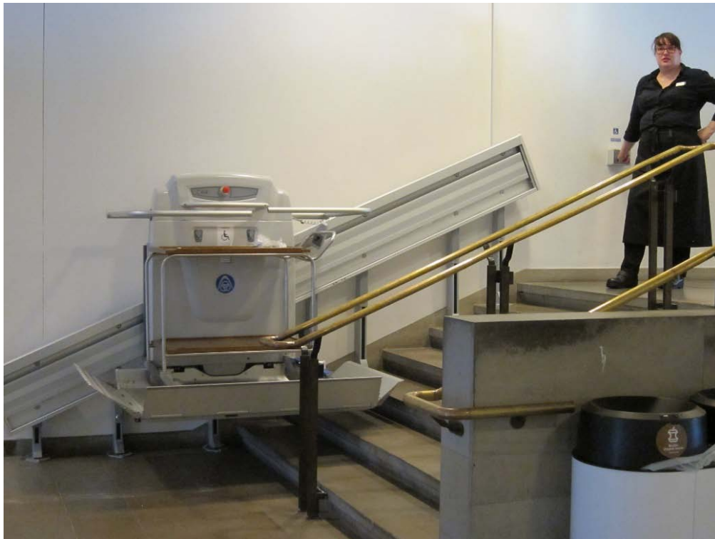
Figure 16. Stair lift in the main lobby, Y wing. Aalto University/Antti Raike.
