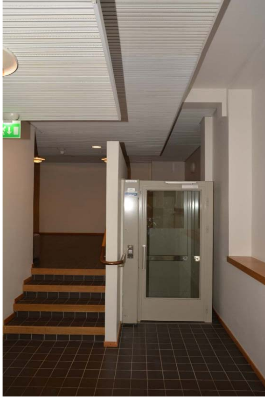
Figure 15. Stair lift in U wing. Aalto University/Jarmo Tiirikainen.
